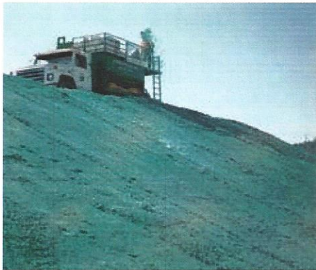
Forms an erosion-resistant, built-in-place blanket that prevents polymer leaching and dispersion of soil particles
